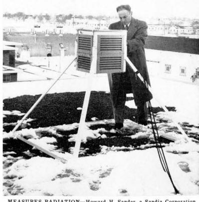
MEASURES RADIATION-Howard H. Sander, a Sandia Corporation engineer in the Weapons Effects Department, 5110, stands beside the instrument which helped measure radiation fallout from the 1955 test series in Nevada. The device showed that the total dose increase of background radiation in Albuquerque amounted to about the same one would receive by wearing a radium dial wrist watch for a year.
